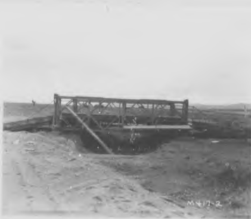
Before ↑ Bailey Bridge. Note: Loose ramp and broken walkway After ↓
